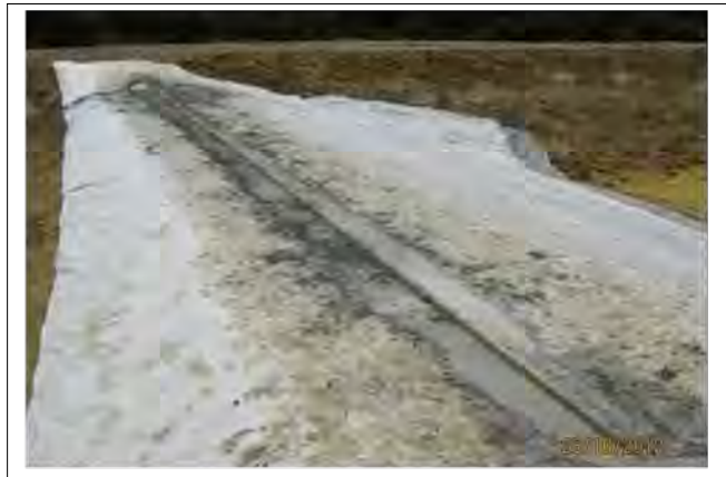
EXAMPLE OF A LEVEL SPREADER
